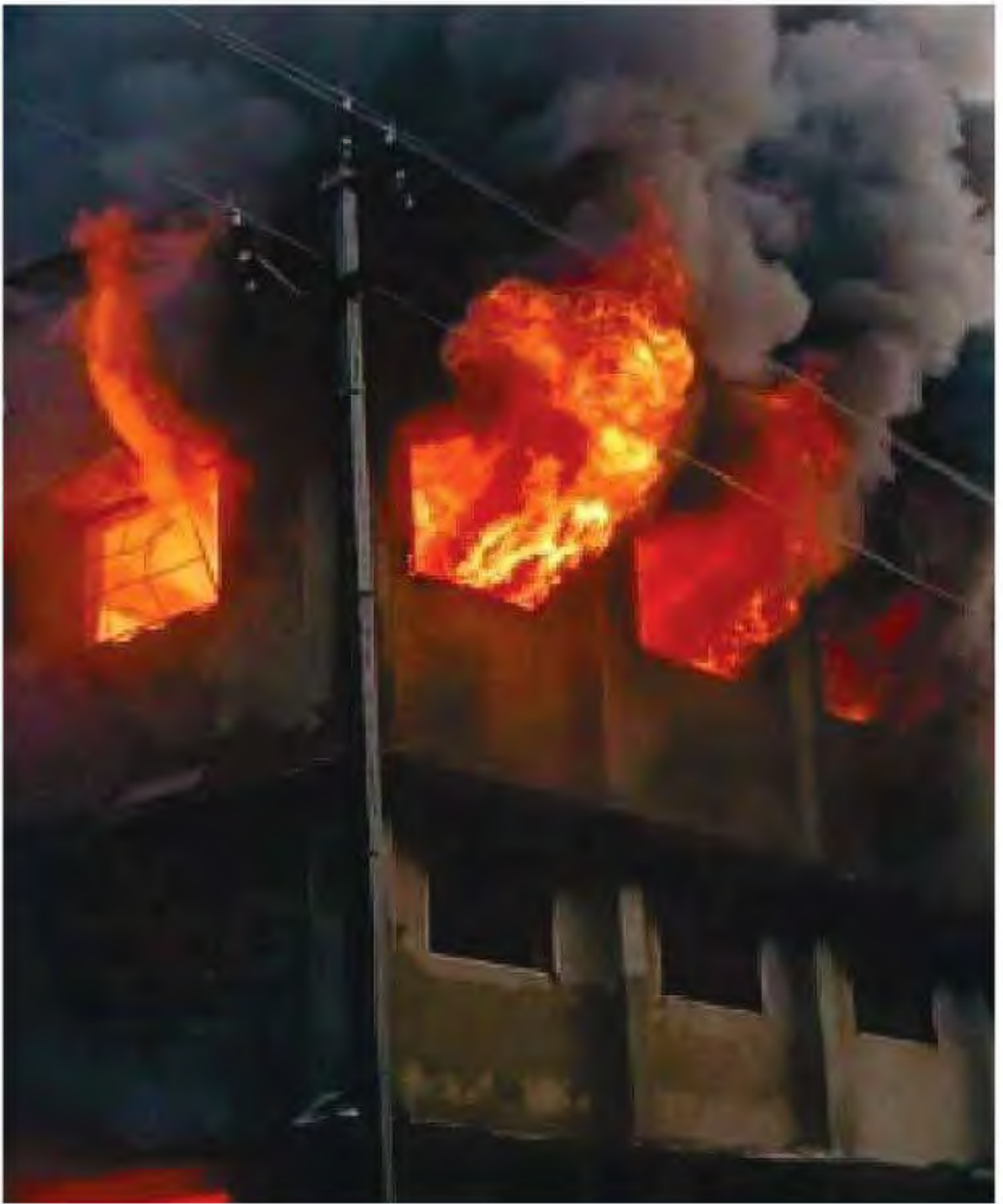
The fire that gutted Gratex House, Navi Mumbai
