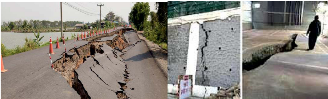
Fig. 9.9: The wide gaps caused by tearing apart roads, floors of the houses, etc.
